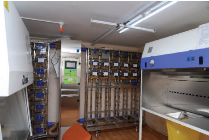
IVC cages and Bio Safety Cabinet
